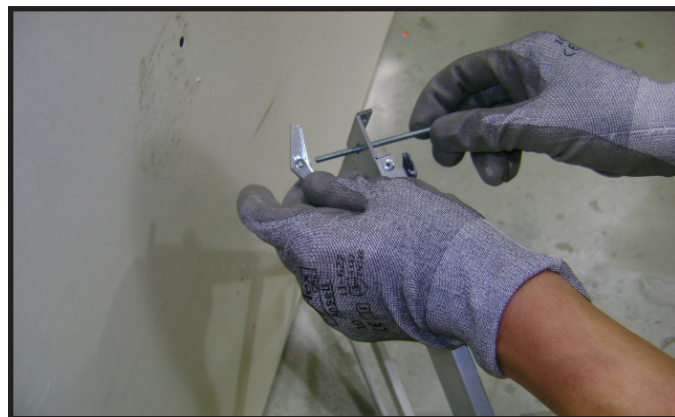
Figure 5 Toggle Bolt Installation through Mounting Bracket
