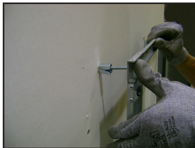
Figure 6 Installing Anchors in Hollow Wall
